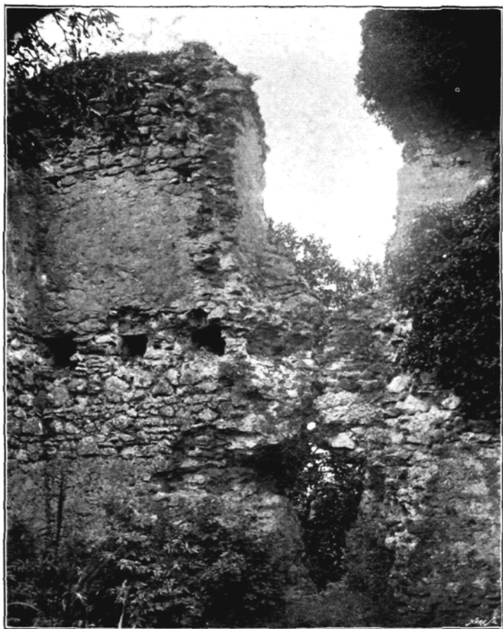
INTERIOR FROM NORTH-WEST CORNER, SHEWING PRESENT GROUND LEVEL AND BEAM HOLES.
